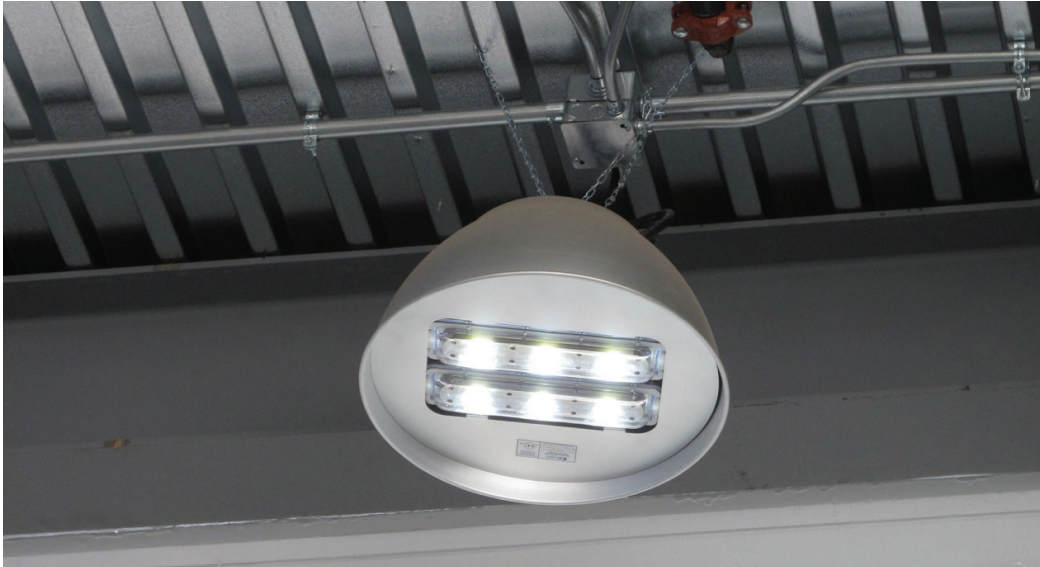
LED lighting installation in storage area
