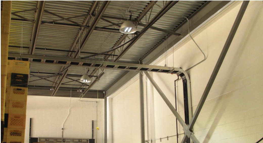
LED lighting installation in storage area
